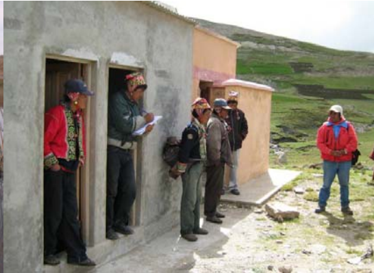
Construction of bathrooms in Kalachaca
